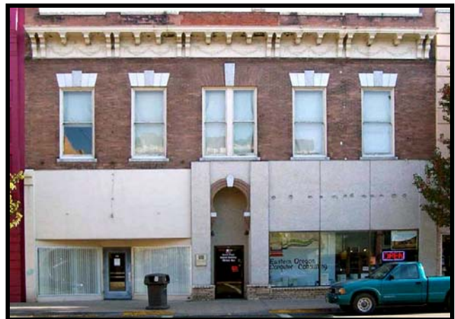
La Fontaine Building, Pendleton, OR
